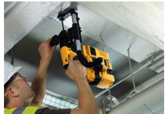
Rotary hammer with built-in VDCS including HEPA filter. Note the shroud, hose and vacuum.
